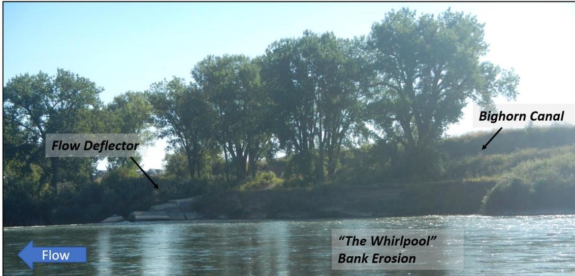
Figure 19. View across river showing severe bank erosion upstream of a large concrete flow deflector.
