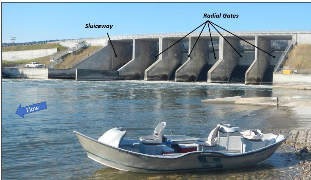
Figure 16. View upstream of Afterbay Dam showing five radial gates and sluiceway (09/05/2019, ~3,200cfs).
