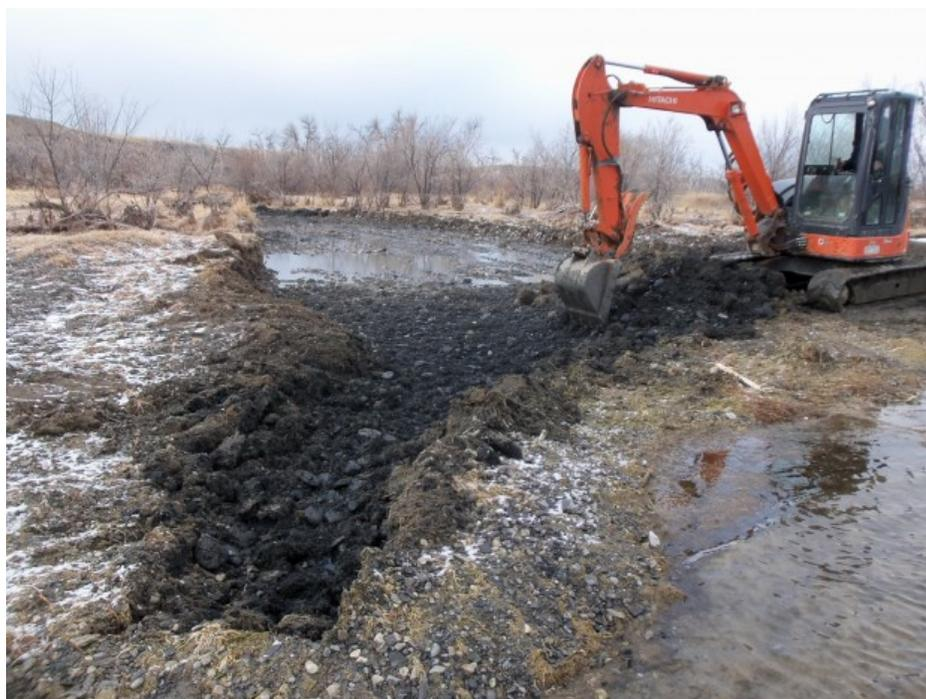
A mini-excavator is used to remove gravel from the head of a Bighorn River side channel to restore the water flow.
